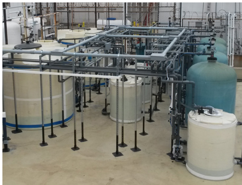
A MAC-based Toxsorb system for the removal of chrome and cyanide in an electroplating facility in California.
