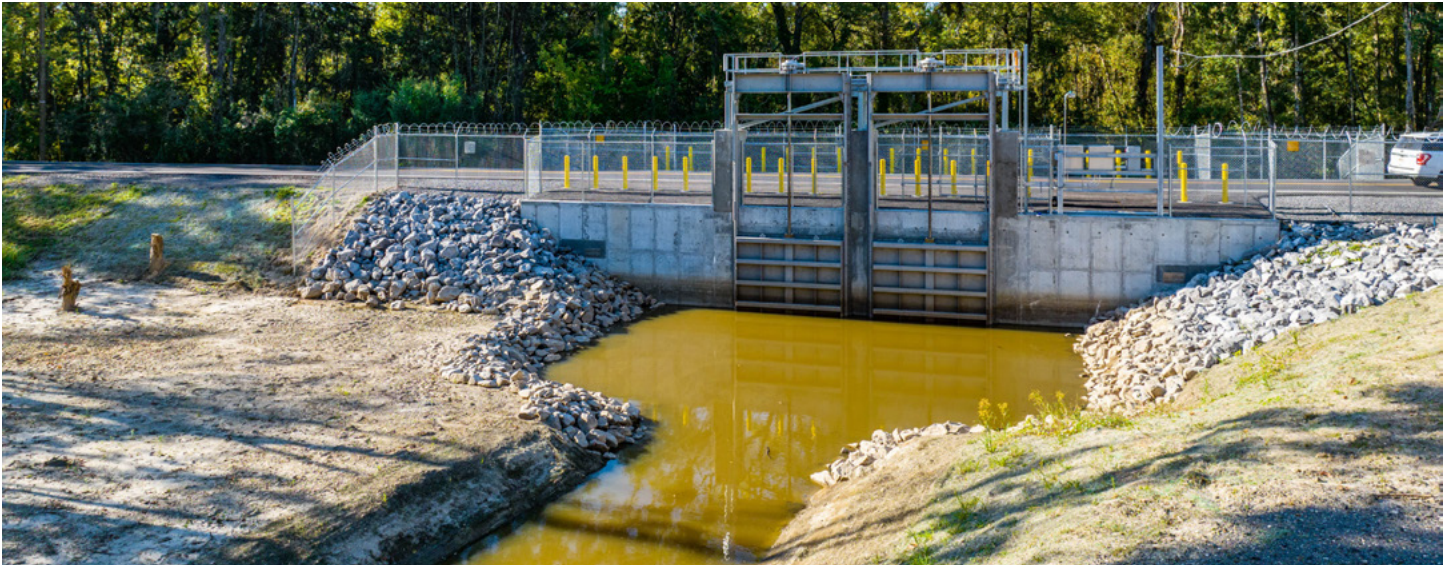
McKim & Creed built two SCADA-controlled gated control structures to help reduce flood risk for the Pontchartrain Levee District of Ascension Parish, Louisiana.
