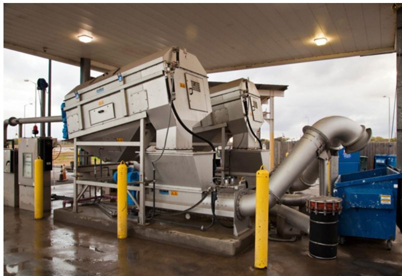
HUBER's RotaShield is a trailer that takes septic waste directly from haulers and removes the solids before that waste goes into a wastewater treatment plant.
