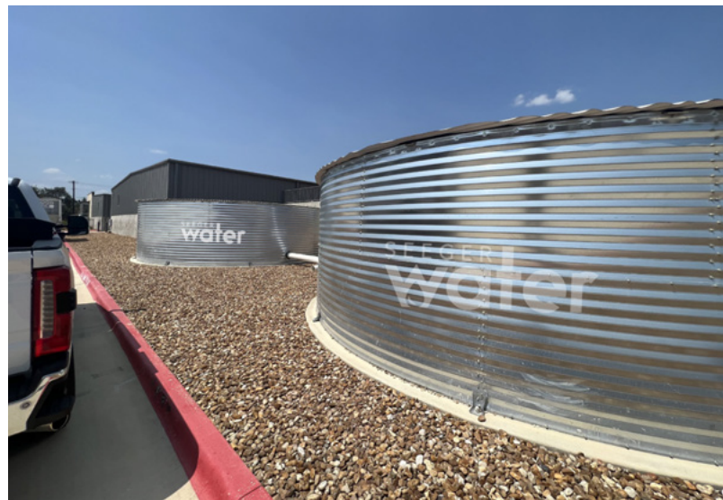
These tanks form part of a rainwater recycling project that stores and cycles 150,000 gallons of rainwater for irrigation.
