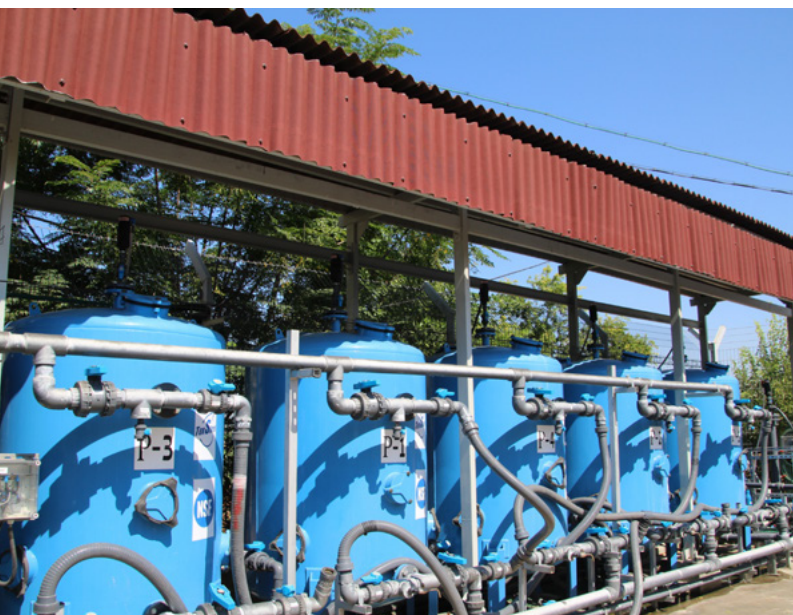
A MAC-based Toxsorb system for removing perchlorate from ground water that will be used as drinking water in Israel.
