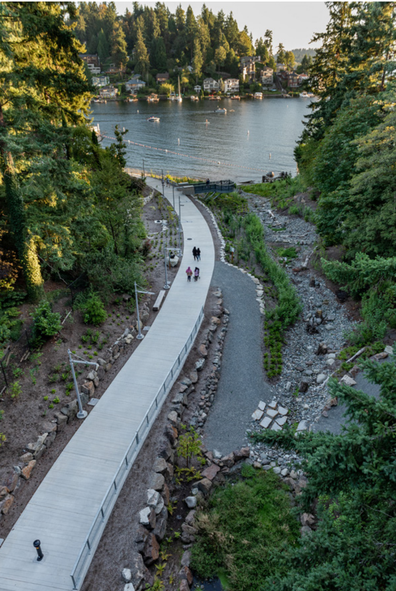
In Meydenbauer Bay Park in Bellevue, Washington, a 300-foot-long restored stream channel (left) replaces a buried storm water outfall that drains a large urban area to Lake Washington, improving water quality and habitat. An open, cobble-lined channel (right) conveys treated storm water from a new parking area to infiltration facilities adjacent to Lake Washington.
