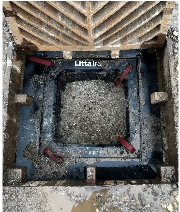
A LittaTrap placed in a catch basin near a loading dock. The LittaTrap has captured thousands of tiny resin nurdles, which can easily wash into waterways.
