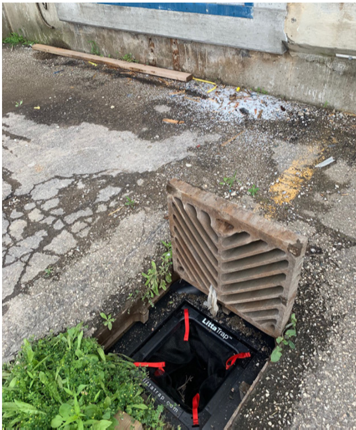
A LittaTrap placed in a catch basin near a loading dock. The LittaTrap has captured thousands of tiny resin nurdles, which can easily wash into waterways.
