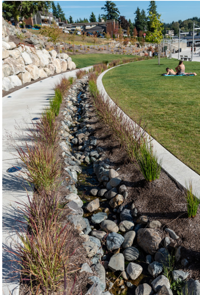
In Meydenbauer Bay Park in Bellevue, Washington, a 300-foot-long restored stream channel (left) replaces a buried storm water outfall that drains a large urban area to Lake Washington, improving water quality and habitat. An open, cobble-lined channel (right) conveys treated storm water from a new parking area to infiltration facilities adjacent to Lake Washington.
