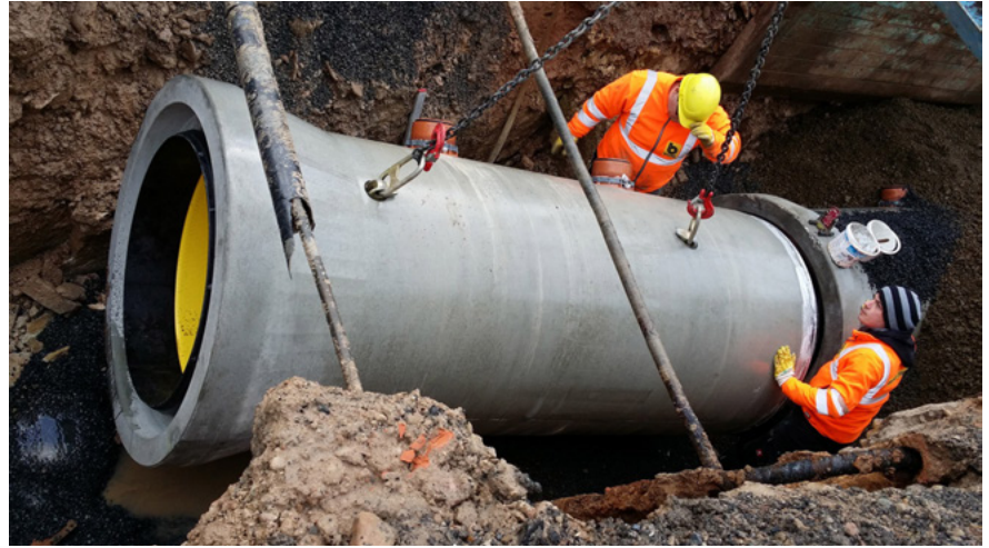
Perfect Pipe and Perfect Lined Manhole feature a joint design that eliminates the need for field welding in most diameters. This saves time and money in the installation process and ensures a quality connection. Perfect Pipe is ideal for open-trench or trenchless installation and performs well in high-water-table environments.
